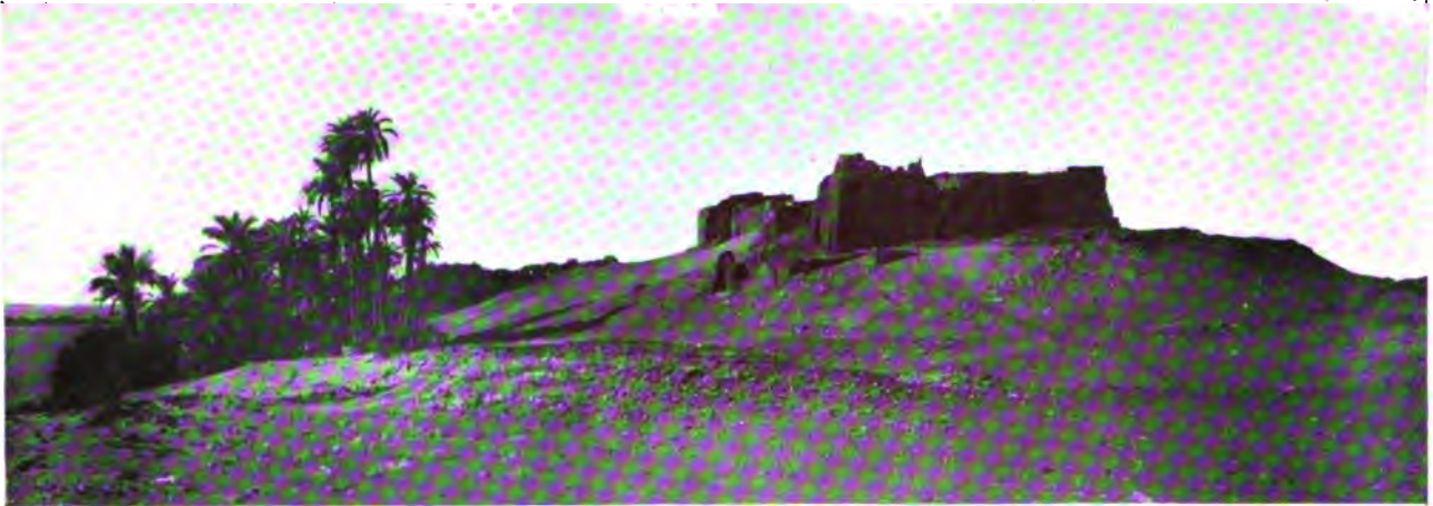
(a) The central building from the north.
